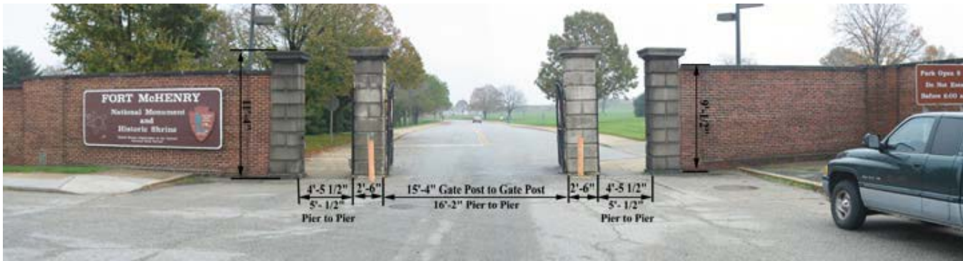
Figure 13 Dimensions of the entrance gate.
