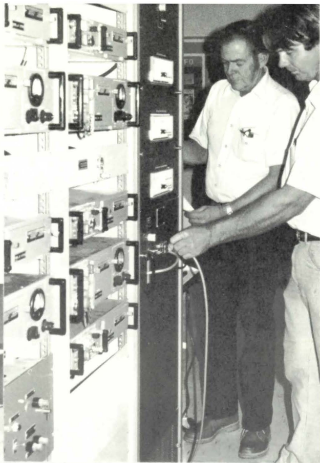
A--Drew Stallings (left), Electronic Supervisor, and John Farmer, Airway Facilities Technician-In-Depth, at the Remote Maintenance Control (RMC) (second generation Lake Tahoe VORTAC) which automatically monitors and checks navigational aids to ensure proper operating equipment for pilot safety.
