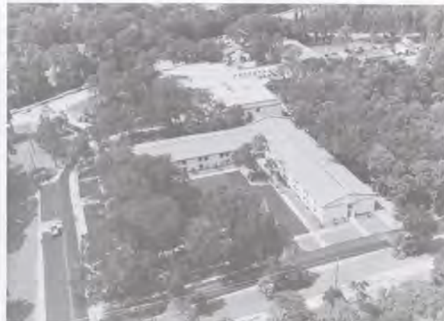
Aerial view of FAA's Center for Management Development, which is located in a wooded area at Palm Coast, Florida, north of Daytona Beach.
