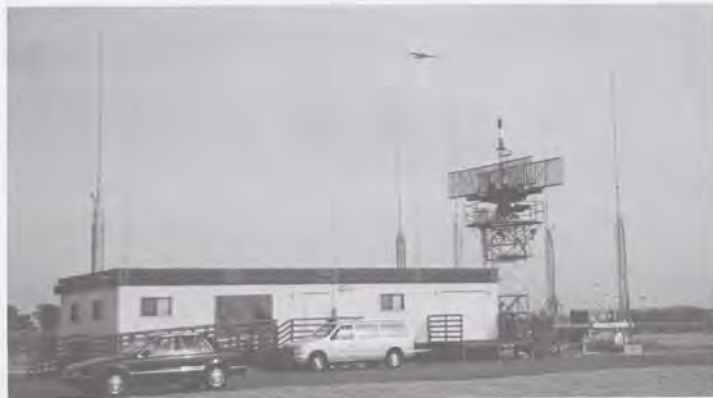
The test facility at Memphis shows the back-to-back Mode 5 or secondary radar antenna. The displays are in the trailer where the test exercises are run.
