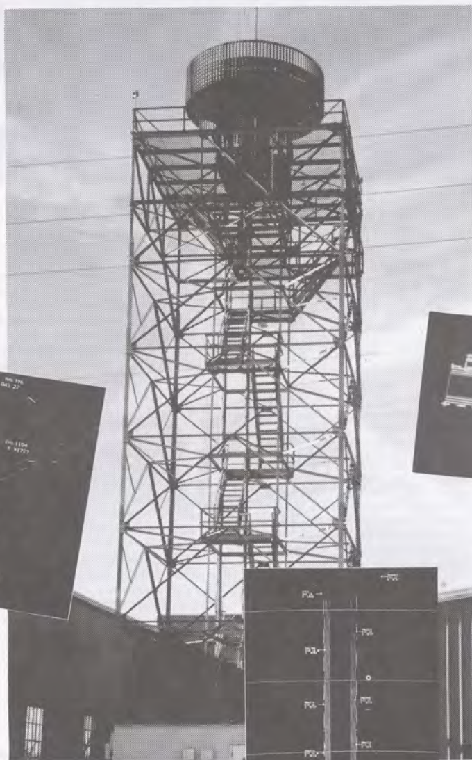
This electronic scanner antenna is at Raleigh-Durham, one of the two PRM test sites. It provides target updates to the controllers every second or faster.
