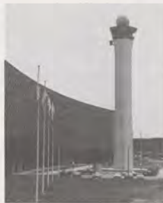
Chicago O'Hare International Airport Air Traffic Control Tower.
