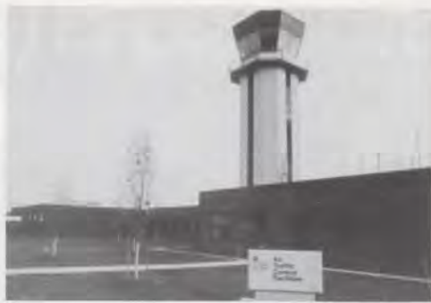
The unique facility at Burlington, VT, is composed of a tower base building (at right), an AFSS (at left) and a tower joined together by a glassed-in walkway. The tower itself rises to 95 feet above ground. Controllers in the cab work at the 77-foot level.
