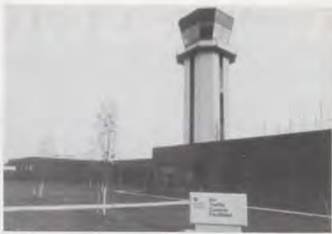
The unique facility at Burlington, VT, is composed of a tower base building (at right), an AFSS (at left) and a tower joined together by a glass-enclosed walkway. The tower itself rises to 95 feet above ground. Controllers in the cab work at the 77-foot level.
