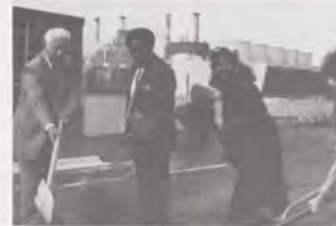
Central Region's Freddie Thompkins (second from left) helped break ground for an all-new day care facility in the Bannister Federal Complex in South Kansas City.
