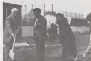
Central Region's Freddie Thompkins (second from left) helped break ground for an all-new day care facility in the Bannister Federal Complex in South Kansas City.
