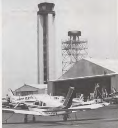
The Quick Scan radar tower is a close neighbor to the airport control tower. The bright red circular radar measures 17 feet in diameter.
