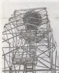
Seventy-seven feet of steel reach skyward at the Raleigh-Durham Airport to cradle the high tech Quick Scan radar.
