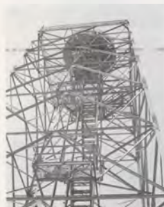
Seventy-seven feet of steel truss skyward at the Raleigh-Durham Airport to cradle the high tech Quick Scan radar.
