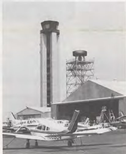
The Quick Scan radar tower is a close neighbor to the airport control tower. The bright red circular radar measures 17 feet in diameter.
