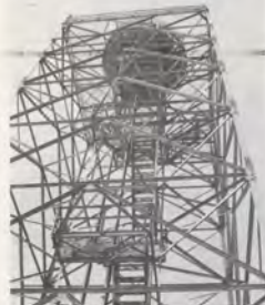
Seventy-seven feet of steel reach skyward at the Raleigh-Durham Airport to cradle the high tech Quick Scan radar.
