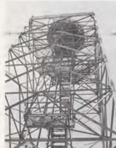
Seventy-seven feet of steel reach skyward at the Raleigh-Durham Airport to cradle the high tech Quick Scan radar.
