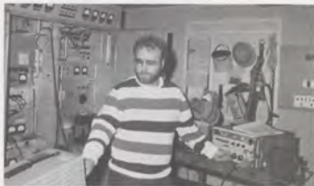
Wilmington, N.C., AFSFO electronics technician Russell Ballard fine tunes the airport surveillance radar.
