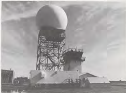
The Deadhorse, Alaska, beacon-only radar—FAA's most northerly unmanned radar, sitting on the Arctic Ocean—can tell the Anchorage ARTCC how it's doing even in the dead of winter when the temperature drops below minus 70 degrees Fahrenheit. It does so through the National Beacon-Only Remote Maintenance System (RMS) prototype, which notifies the center within five seconds of any out-of-tolerance condition at the site.
