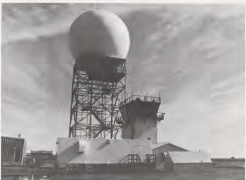
The Deadhorse, Alaska, beacon-only radar—FAA's most northerly unmanned radar, sitting on the Arctic Ocean—can tell the Anchorage ARTCC how it's doing even in the dead of winter when the temperature drops below minus 70 degrees Fahrenheit. It does so through the National Beacon-Only Remote Maintenance System (RMS) prototype, which notifies the center within five seconds of any out-of-tolerance condition at the site.
