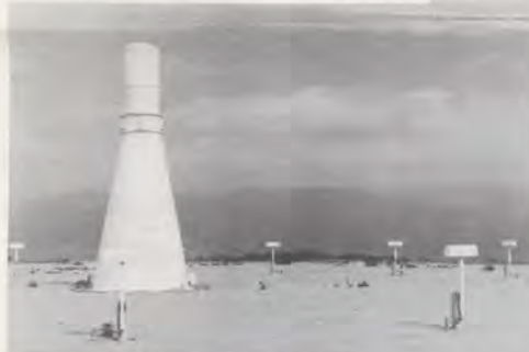
The Fillmore, Calif., VORTAC shows the cone-shaped VOR antenna housing on the ground, surrounded by the cylindrical TACAN antenna, the entire counterpoise ringed by ground-check detectors. The equipment shack is elsewhere.
