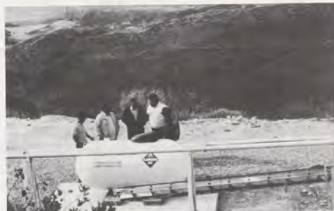
Los Angeles sector technicians discuss some modifications that were needed on the new above-ground propane fuel tank that feeds the backup power generator.
