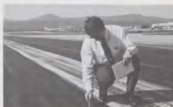
Cimino evaluates tire rubber deposits in pavement grooving for possible removal. The grooving increases friction by reducing water buildup beneath aircraft tires in wet weather.
