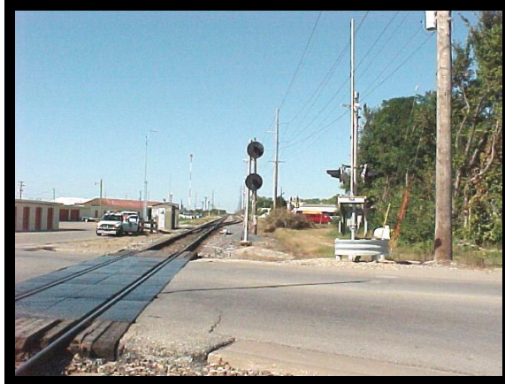
Figure 2. Northeast corner facing west.
