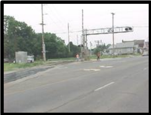
Figure 3. Southeast corner facing northeast.
