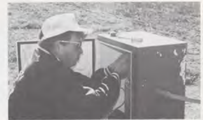
Donald Marlette, maintenance mechanic foreman at the Haron, S.D., SFO's Environmental Support Unit, works on the MALSR flasher (approach lighting) at the Aberdeen, S.D., Airport.
