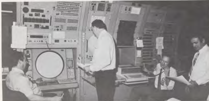
National Airspace System (NAS) managers Eston Shipley (standing, center) and Billy Stephens (right) coordinate facilities shutdowns at the Indianapolis ARTCC with the help of NAS specialists Richard Sitzman (left) and Joseph Kramer.
