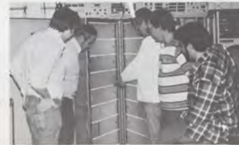
Discussing an equipment cabinet at the Tyler, Minn., SFO are (from the left) electronics technician Dan Schmidt, SFO manager Gudmund Broin, electronics technicians Jon Bloom and Gary Hager and developmental electronics technician Gary Wozniak.
