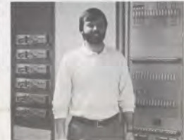
Pausing in his work on ICSS equipment at the Rapid City, S.D., Sector Field Office is electronics technician Larry Burkhead.
