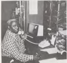
Inter-Facility Data Unit technician Richard Garmay coordinates trouble calls concerning communications equipment.
