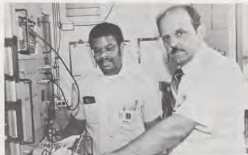
ILS Unit supervisor Frank Salviolo (right) and ILS technician Willie Flowers test the Runway 4R distance measuring equipment.
