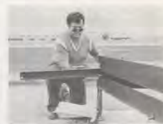
Gene McCarthy checks the level of the Runway 13L VASI (Visual Approach Slope Indicator) Box.
