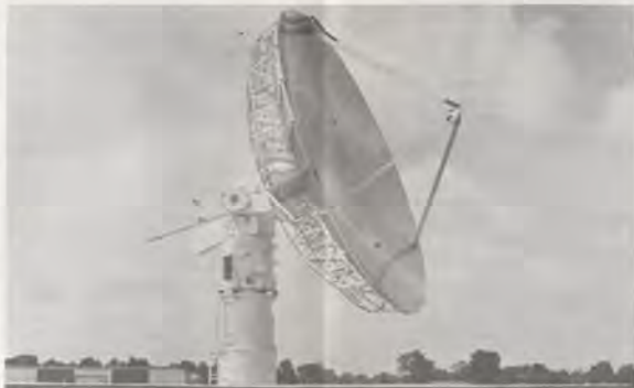
An earlier FAA NEXRAD test bed for both terminal and enroute configurations placed this 30-foot parabolic antenna at Olive Branch Airport, 10 miles from Memphis, Tenn., International Airport, in 1984.
