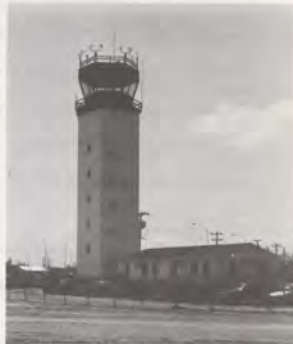
Providence's tower is a modular, turnkey type with a separate base building.
