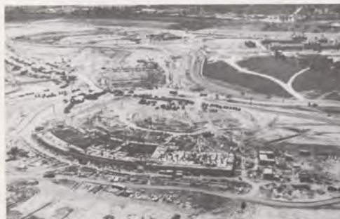
The entire area east of the George Washington Memorial Parkway in northern Virginia was just a bare plain as the terminal was being constructed in 1940. Most of where the airport stands was sand and gravel fill in the Potomac River.
