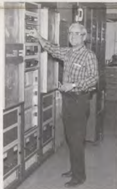
Harry D. Cunley, communications electronics technician, checks the performance of the multi-channel recorders at the Albuquerque Center.
