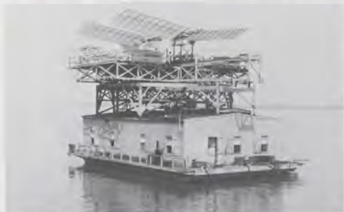
Langley's Aerodrome attempted flight in October and December of 1903, but fouled on its launchers both times, ending up in the Potomac River.
