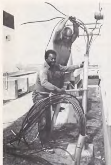
Resident engineer Les Thomas (foreground) and marine machinery mechanic Phil Bourgeois run cables to the standby engine generator at the New Orleans Lakefront tower under construction.
