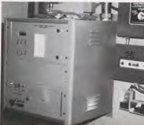
Another configuration of a Remote Monitoring Subsystem is this portion of one that services a long-range radar.
