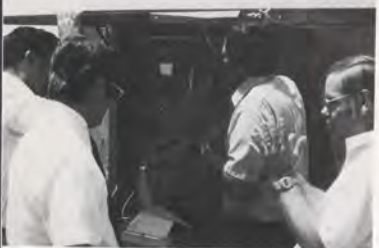
Central Region Airway Facilities personnel examine the installation of a Remote Monitoring Subsystem that tends landing lights at the Johnson County Executive Airport in Olathe, Kan.
