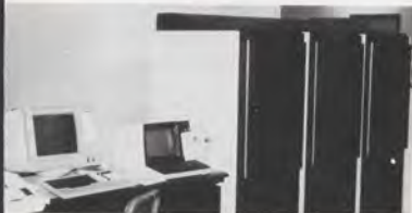
The workhorse of RMM is the Maintenance Processor Subsystem—the computer that queries the facility, processes its data, stores it and takes remedial instructions back to the facility.
