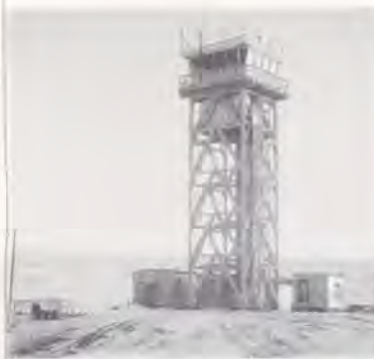
On the barren top of the world stands the control tower at Thule Air Base.
