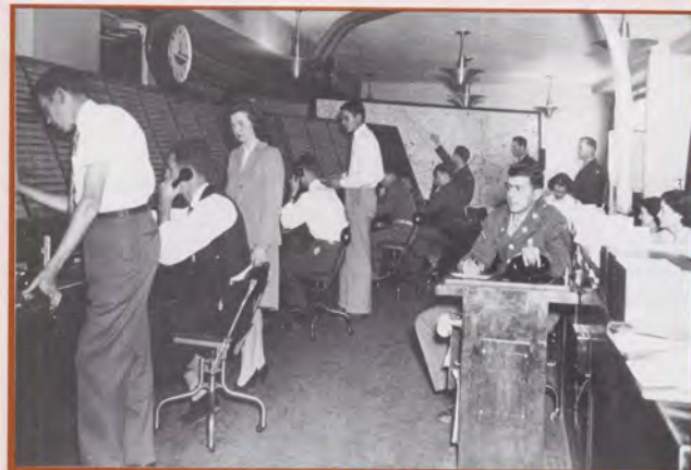
In November 1943, the Washington National Airport Airway Traffic Control Center was a first-generation facility. The presence of women and soldiers marks this as a wartime setting.
