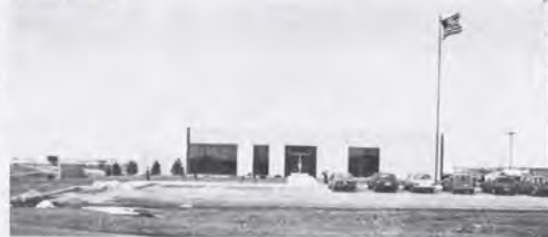
The Bridgeport AFSS's new building typifies the new automated station.
