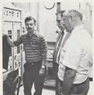
Electronics technician Herb Pearce (left) shows some of the Fort Lonesome equipment to Airway Facilities Division assistant manager Don Davis and Southern Region Director Jonathan Howe (right).
