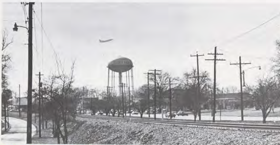
This College Park, Ga., water tank was deemed a hazard to traffic at Hartsfield International Airport, the major terminal for Atlanta. It was torn down as soon as a new one was built elsewhere.
