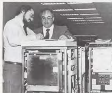
Sperry personnel make notes while performing equipment verification during installation testing.
