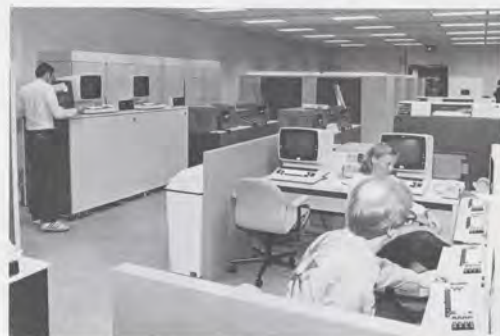
During a nighttime installation session, IBM engineers in work clothes begin system diagnostics at terminals like those that will be used at supervisors' work stations in en route centers.
