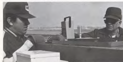
Electronics technicians Dale Engelhaupt (left) and Jack Schaeffer perform maintenance on the Chadron visual approach slope indicator (VASI).
