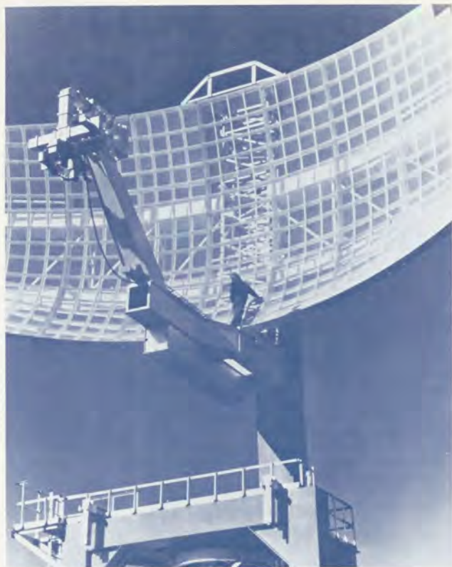
Today's long-range radar is the ARSR-3, which was introduced in 1977.
