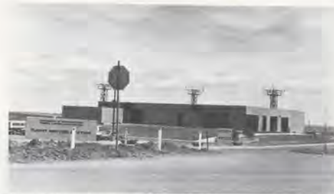
Opened this spring, one of the agency's 61 automated flight service stations graces the Arapahoe Airport.
