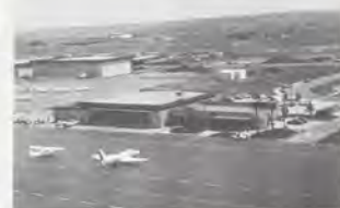
The existing Combs-Gates terminal.
