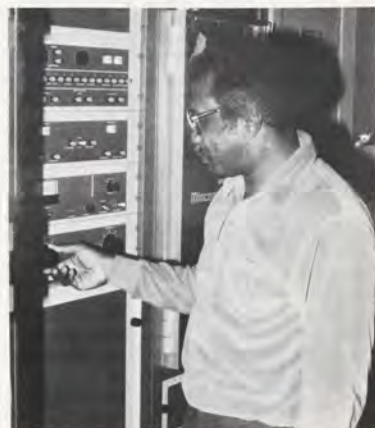
Making an adjustment on a system monitor is communications technician James Brown.
