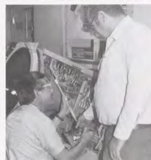
Electronics technicians Dick Fong (left) and Arlie Williams of the Oakland ARTS Sector Field Office repair a maintenance console at the Oakland Bay TRACON.
