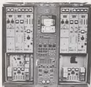
An old VORTAC. All of the tube-type monitoring equipment in both the left and right equipment racks are contained behind the blank panel in the top section of the solid-state TACAN rack, at left in the photo at the right.
