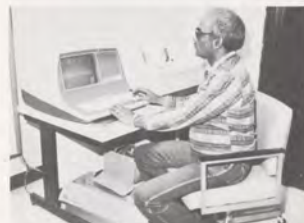
Environmental technician Henry Harris makes a routine check on the computer monitoring system (CCMS) at the Atlanta Hartsfield International Tower.
