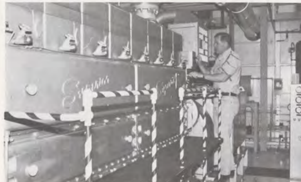
Environmental technician Walt Zarkowski adjusts one of the center's four diesel generators.
