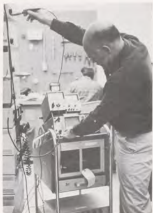
A general NAS sector like Atlanta has many facilities to worry about. Here, electronics technician Charlie Johnson of the Marietta Sector Field Office checks the microwave link for the ASR-8 airport radar at Dobbins AFB.
