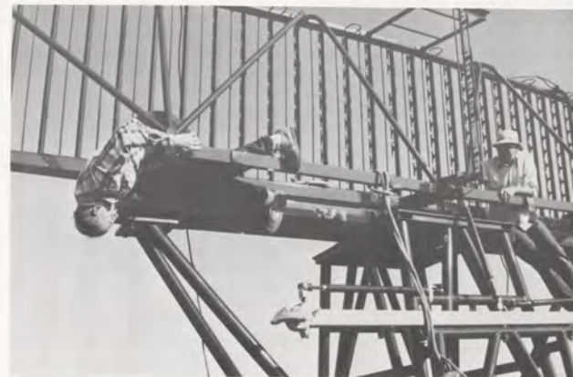
The five-foot open array on Biorka Island is a beacon-only radar for en route identification of transponder-equipped aircraft.
