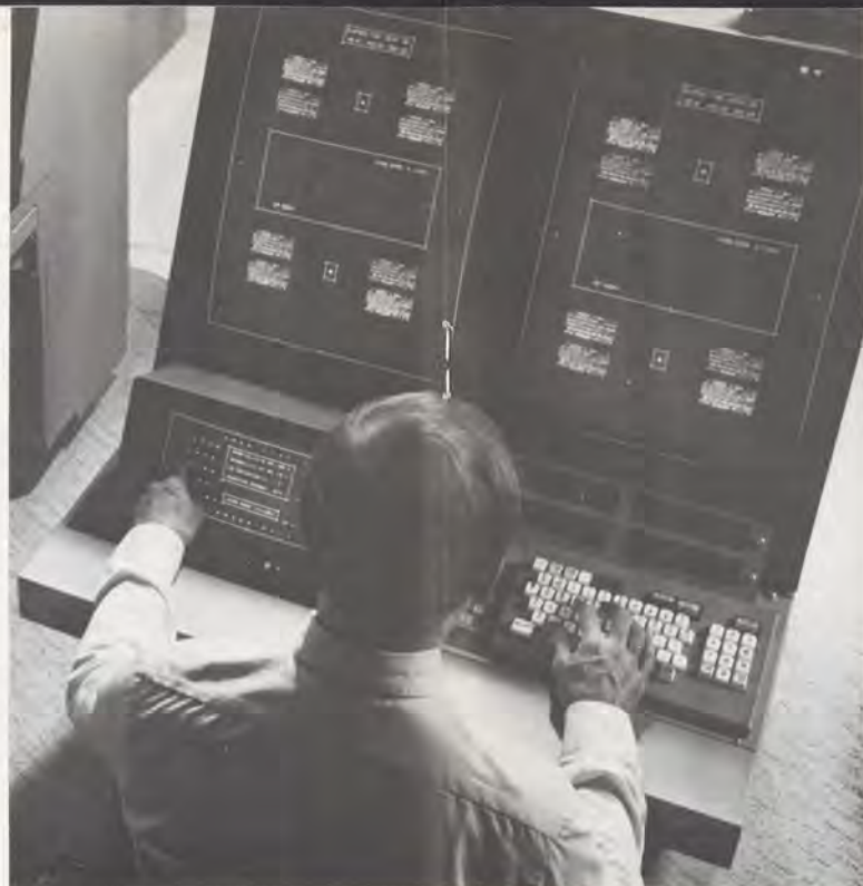
The flight-planning screen might show horizontal and vertical profiles of aircraft, as above, to compare, say, conflicting flight plans.
