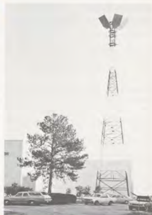
Radar microwave links can be converted to provide interfacility communications in addition to radar remoting.
