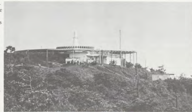
A doppler VORTAC on Taboga Isle, Panama. All are being converted to solid-state.
