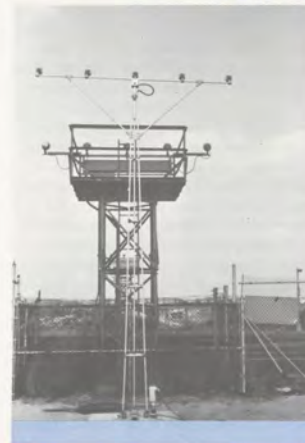
A doppler VORTAC on Taboga Isle, Panama. All are being converted to solid-state.
