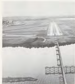
Improvements to approach lighting systems will make them switchable when visibility permits to effect energy conservation.
