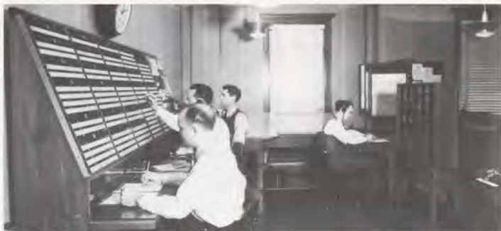
Progress beyond the beginnings: Flight strips are in evidence at the St. Louis airway control station in 1948, here manned by (left to right) John Knoell, Cleon Freeman, Charlie Cliff and Charlie Carmody.
