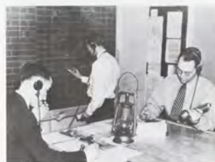
Backup emergency lighting was not very sophisticated in the early centers.
