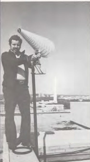
ET Paul Baker installs a conical log-spiral antenna on the roof of the FAA headquarters building. It's used to monitor communications interference.
