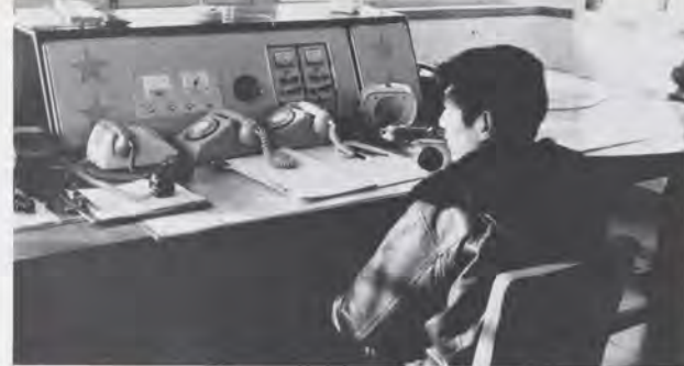
Beijing controller Chen Yong Ming mans a position that provides him with only one communications frequency plus an emergency backup.
