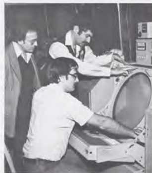
Assistant sector manager Vincent Laurentino (left) checks on ARTS supervisor Tom Gassert (standing) and technician Angus Wall aligning the ARTS IIIA display in the TRACON's computer room.
