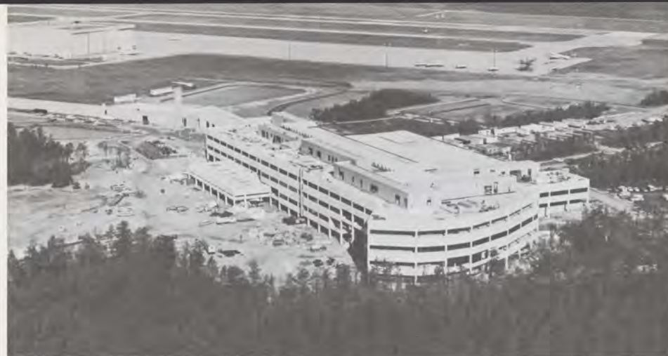
The exterior of the new Technical and Administration Building was almost complete when this photo was taken last fall.
