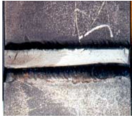
c) Failure surface
