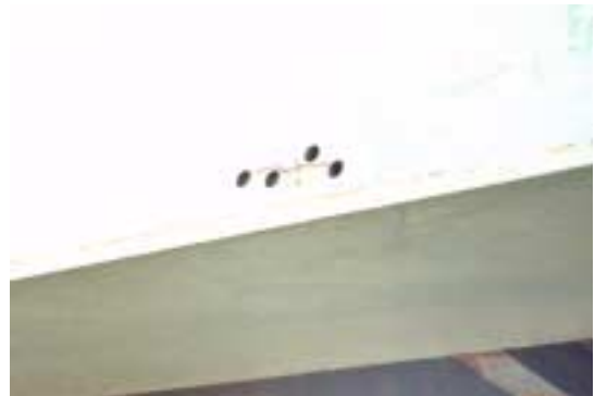
Figure 5.3 Drilled holes used as a crack arrester, at weld connection (left) and two drilled holes for large crack (right)
