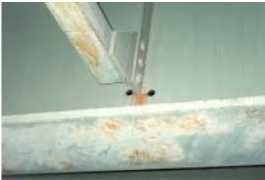
Figure 5.3 Drilled holes used as a crack arrester, at weld connection (left) and two drilled holes for large crack (right)
