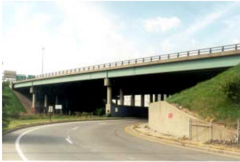
a) Inspected bridge
