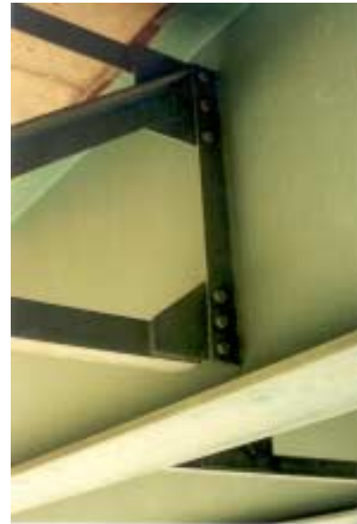
c) The connection between cross frame and girder web
