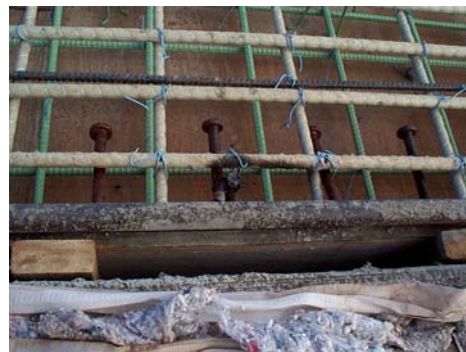
(b) Burned FRP bar due to the use of a flame cutter
