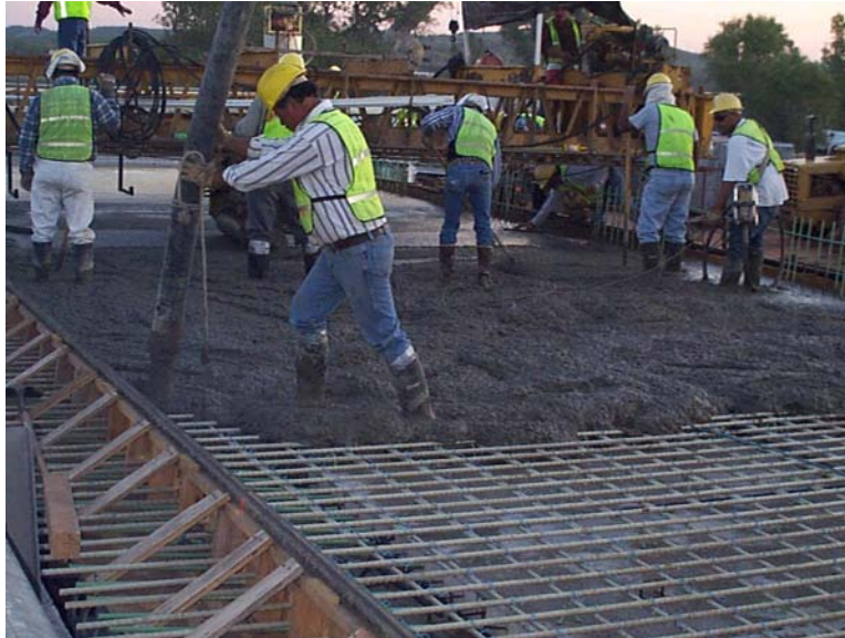
Figure 5.4: Casting Operations (Sierrita de la Cruz Creek Bridge, Amarillo, Texas, 2000)
