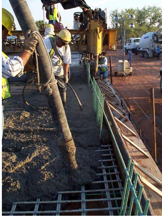
Figure 5.6: Internal Vibrator Compaction (Sierrita de la Cruz Creek Bridge, Amarillo, Texas, 2000)
