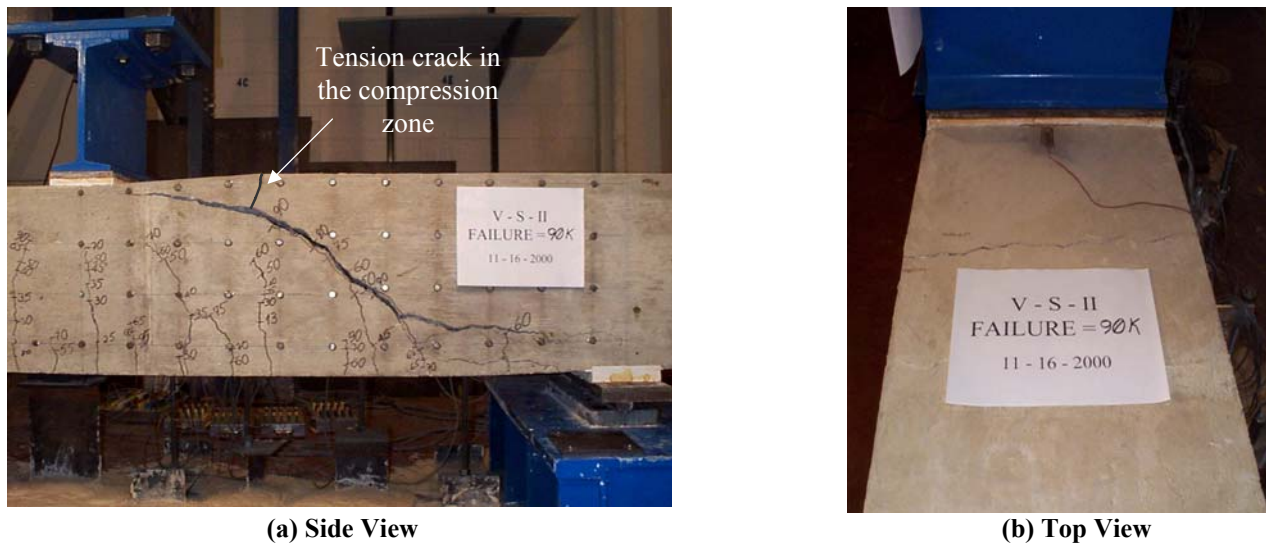
(a) Side View (b) Top View Figure 4.11: Tension Crack on the Top Surface After Failure (V-S-2)
