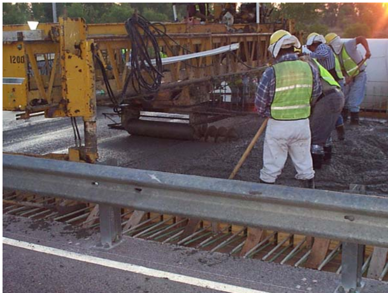
Figure 5.5: Deck Finishing (Sierrita de la Cruz Creek Bridge, Amarillo, Texas, 2000)
