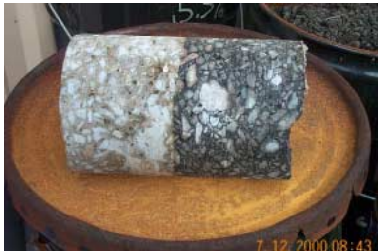
Figure 5.12 Typical UTW core sample taken from the test lanes
