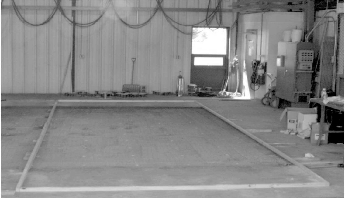
Figure 3.7 Formwork of UTW lanes
