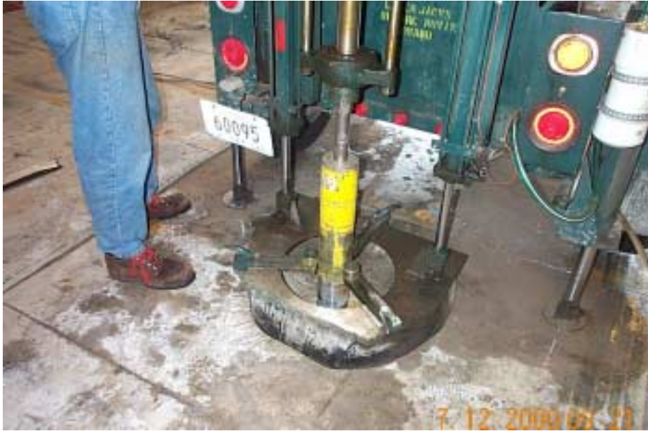
Figure 5.13 Drilling machine removing UTW cores at the APT facility
