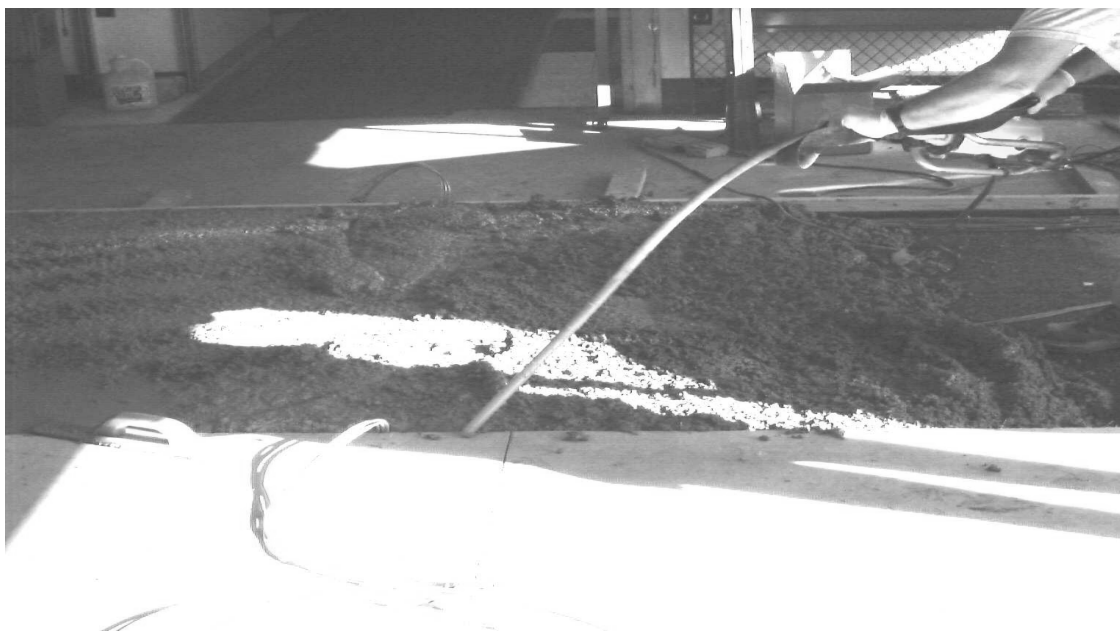
Figure 3.11 Concrete placement at the APT facility
