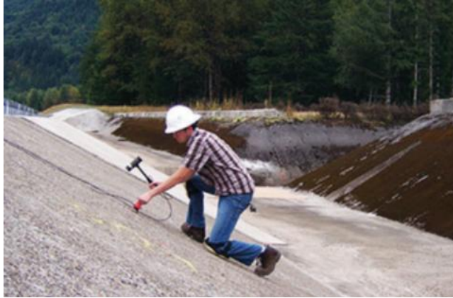
Figure 21 Olson Instruments, Slab Impulse Response
