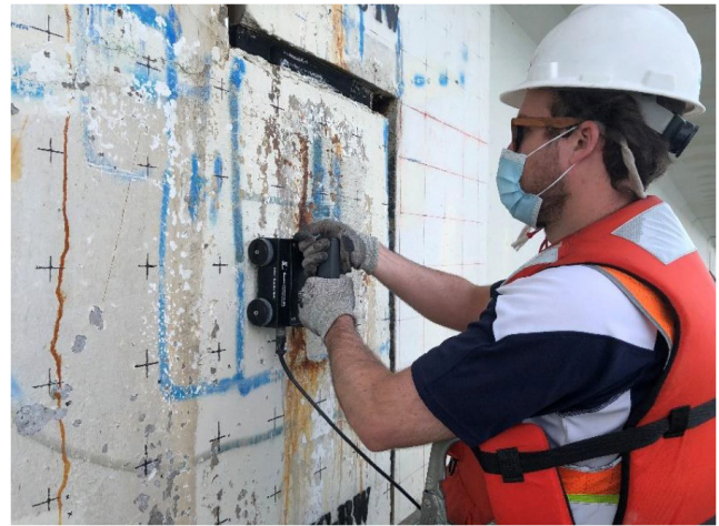
Figure 6.13 Vertical IES on 6-in. Spaced Lines on Bridge Girder (Olson, 2025).
