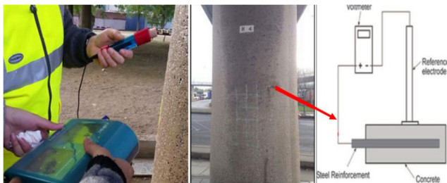
Figure 6.14 Conducting Half-Cell Corrosion Potential Testing.
