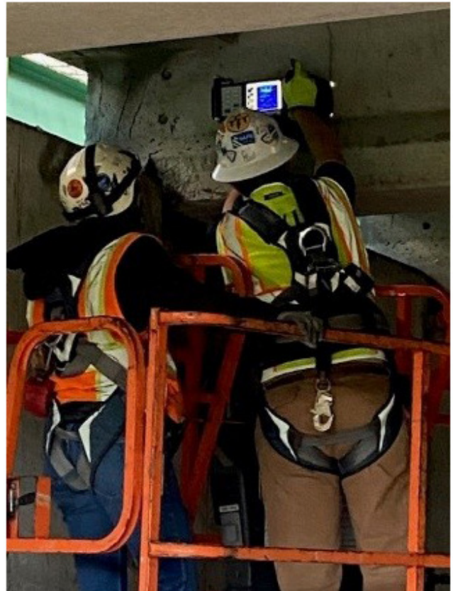
Figure 6.4 Use of MIRA on Concrete Beam End.
