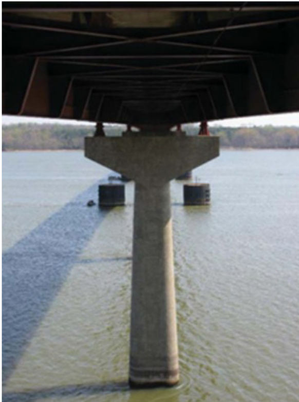
Figure 3.1 RC Pier in John Coffee Memorial Bridge.
