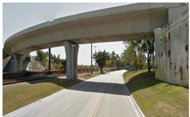
Figure 6.9 Overall View of the Bridge.
