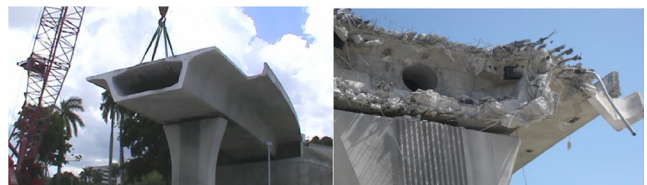
Figure 6.10 Box Girder Cross-Section of the Bridge.
