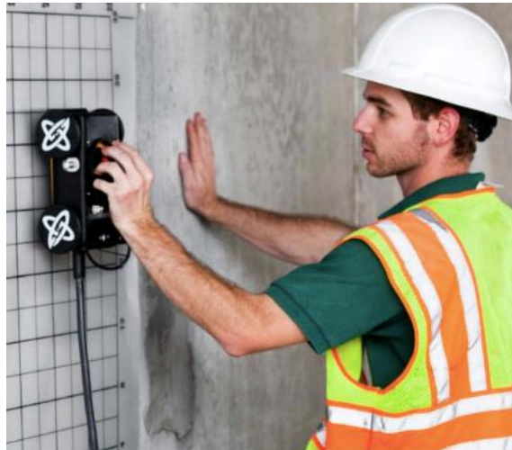
Figure 32 Guideline Geo, Mala ConcreteExplorer / CX System
