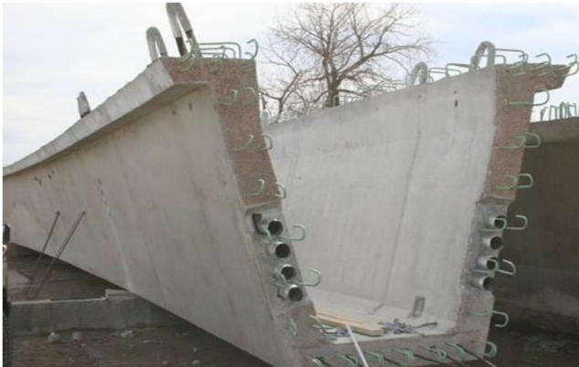
Figure 6.11 Bridge Segment Cross-Section (Olson, 2025).
