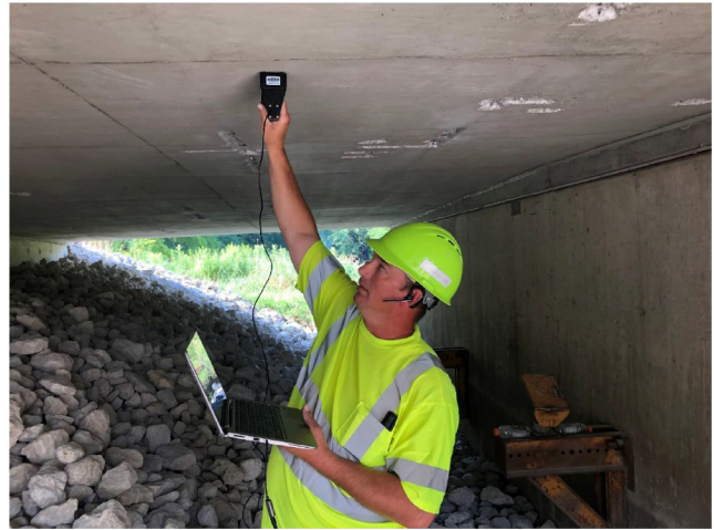
Figure 2.3 IE Testing on a Concrete Bridge Soffit for Thickness and Defect Evaluation.
