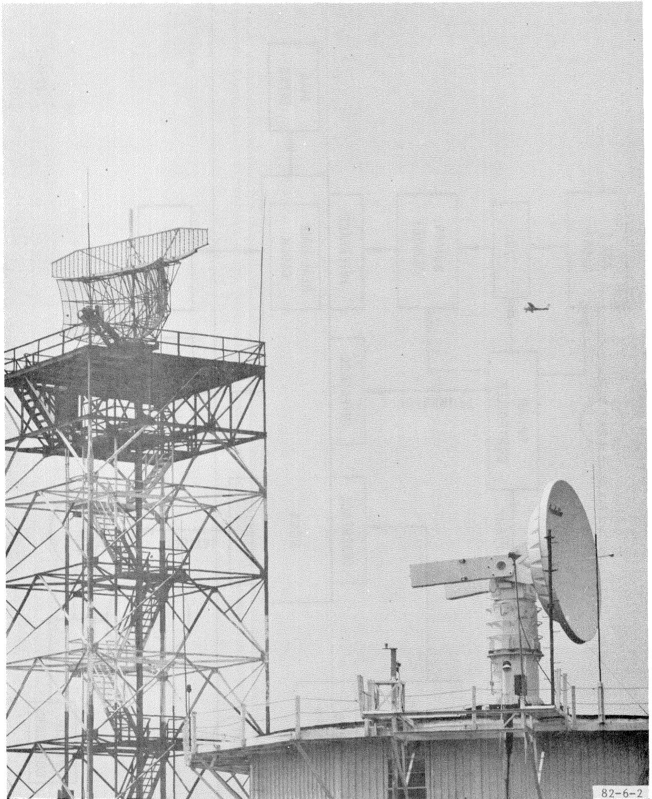
FIGURE 2. ASR AIR TRAFFIC CONTROL AND TURBULENCE ANTENNAS
