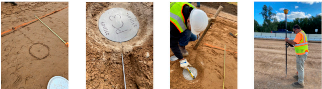
Figure 3.5 Earth Pressure Cell Installation Procedure. Left to Right: Marking Location for Each Sensor, Trench and Ensure Fit, Prepare a Uniform Base for the EPC With Mason Sand, Installing the Sensor and Covering With Subgrade Material. Finally, Each Sensor is Geo-Referenced.
