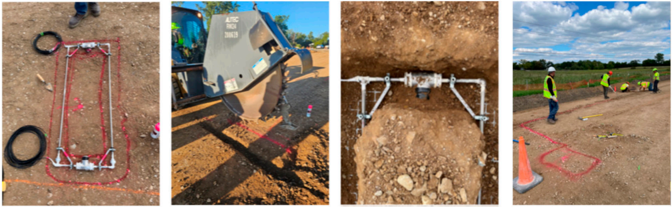
Figure 3.6 BE Field Sensor Installation Procedure. From Left to Right: Mark Location of the Sensor, Prepare Trench, Install the Sensor Frame in Trench Ensuring Uniform Placement Depth, and Finally, fill Sensor and Cable Trenches.
