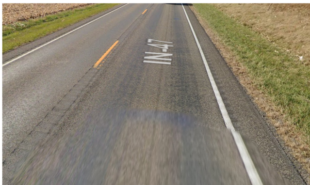
Figure 3.1 Example of Bituminous Concrete Shoulder (Map Image: Google Street View ©).
