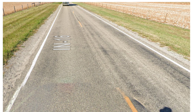
Figure 3.3 Example of Stabilized Shoulder (Map Image: Google Street View ©).
