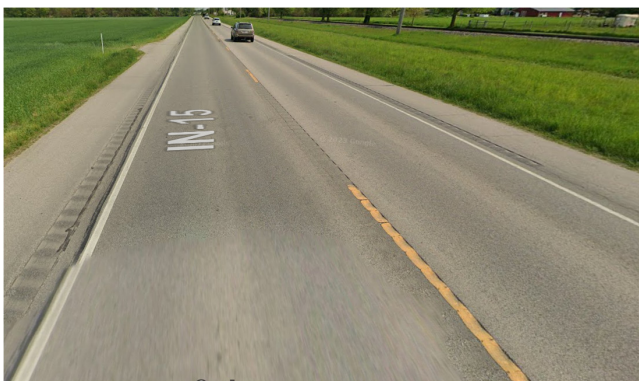
Figure 3.2 Example of Portland Cement Concrete Shoulder (Map Image: Google Street View ©).
