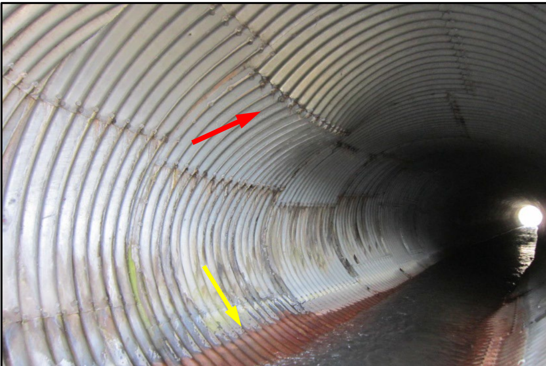
↑ Representative image of the observed sagging in the top panels of the steel plate arch culvert. Deflection estimated at six inches inspected in 2014 (red). Corrosion also apparent at the base of the culvert (yellow).
