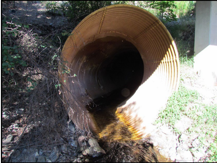
← Overview of inlet of the culvert.
