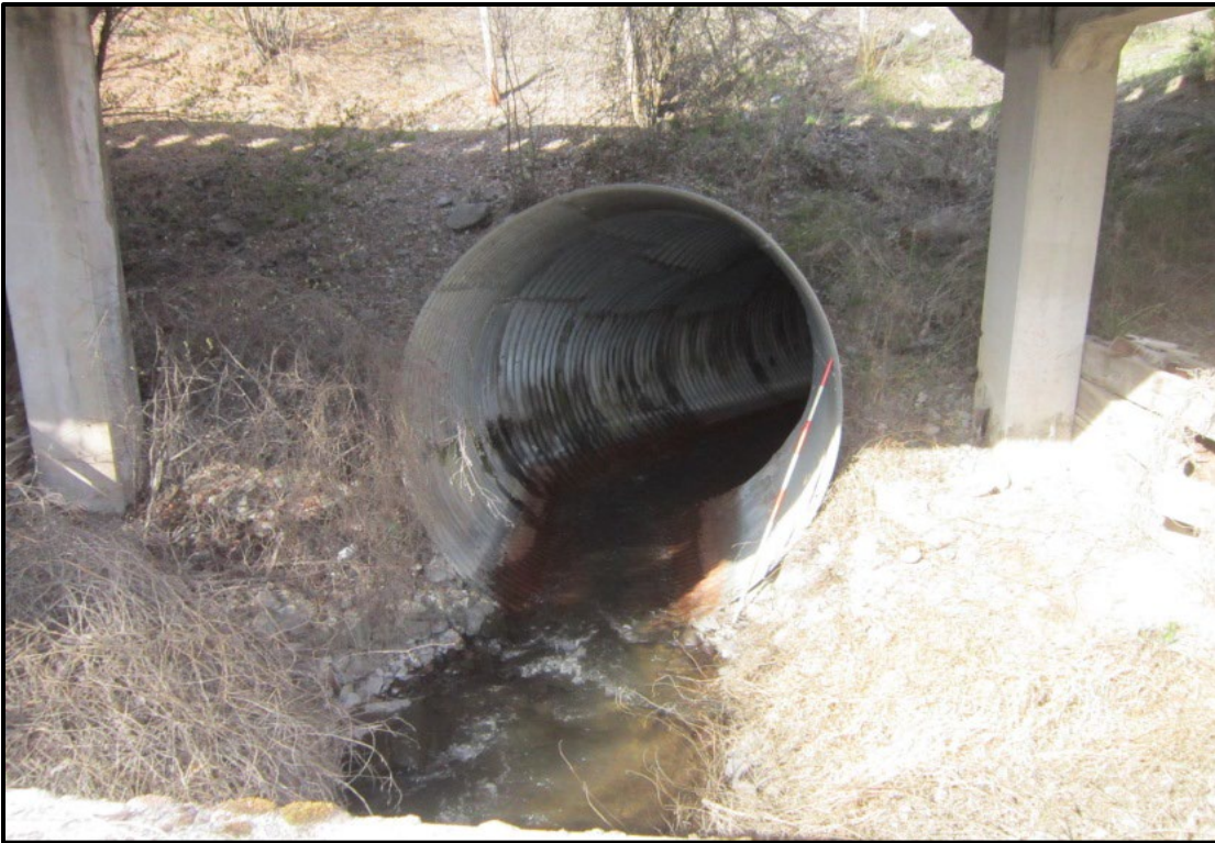
↑ Upstream culvert inlet view, east end.
