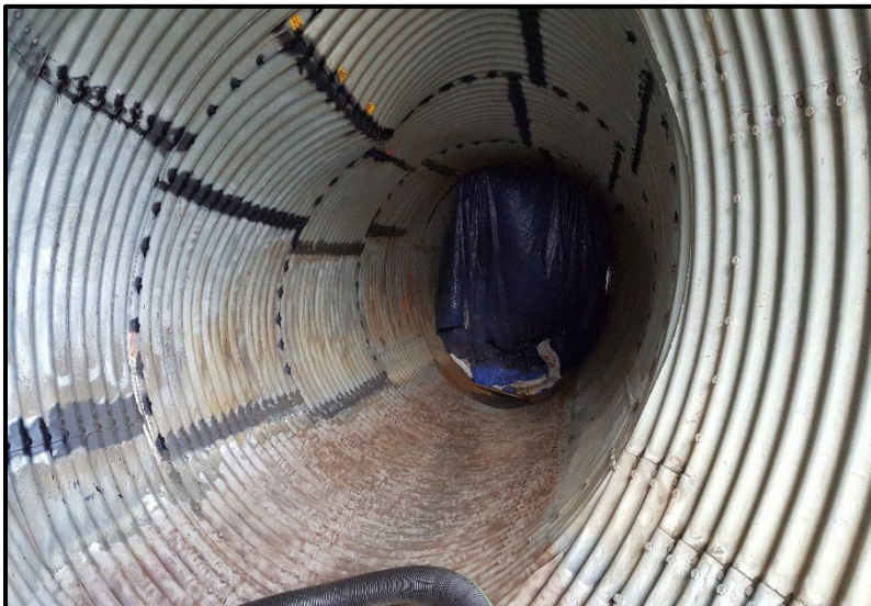
↙ The culvert interior after sand blasting.
