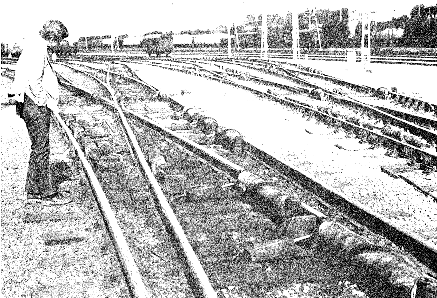
Figure 4-2. ASEA Retarders in Helsingborg Yard
